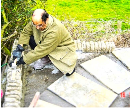
Spirit level is essential, eyeballing can be deceptive on a hill.
